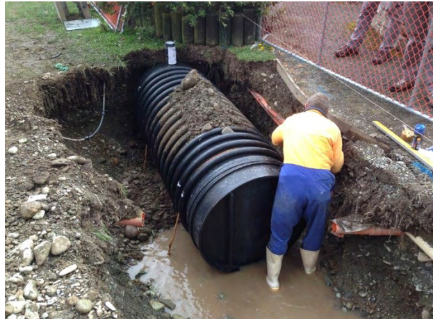
Emergency Holding Tank (2m 3 ) Installation
