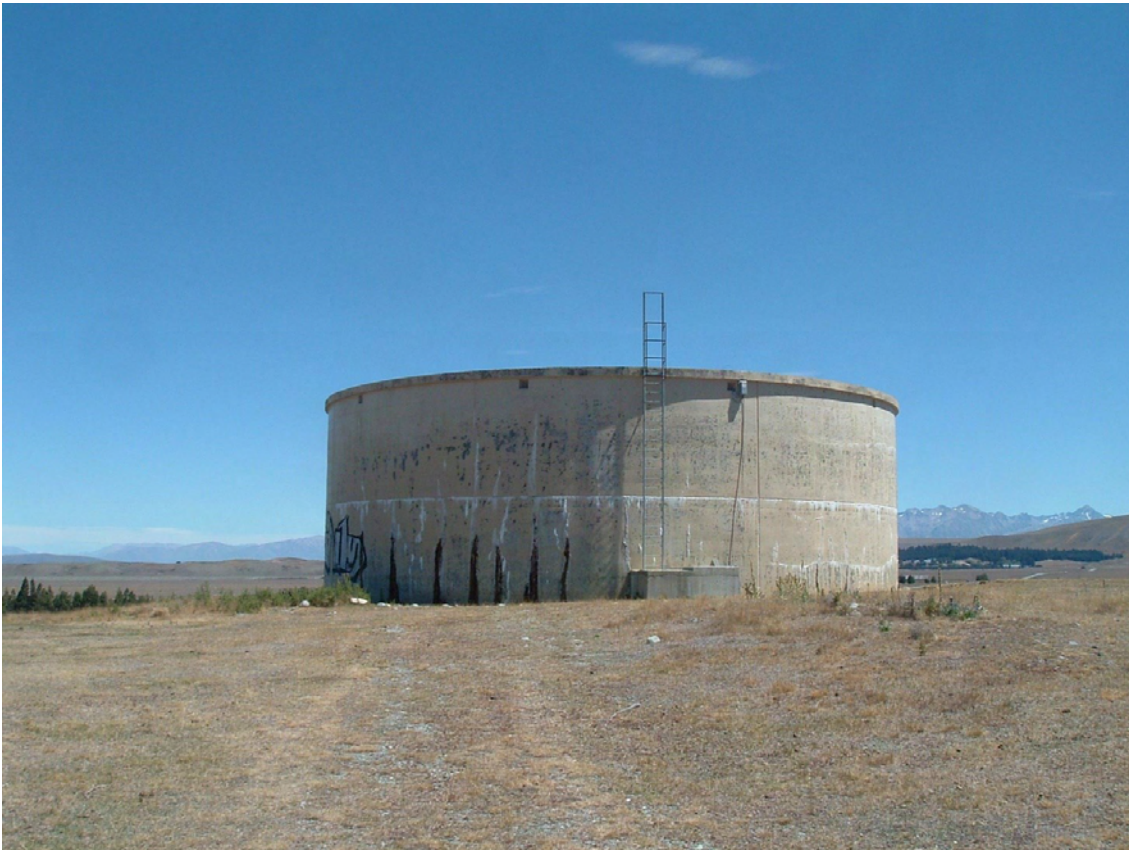
Figure 3.2.4a- Reservoir / Break Pressure Tank
