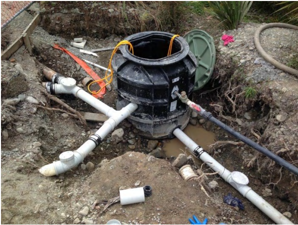
Pump Station Instalation
