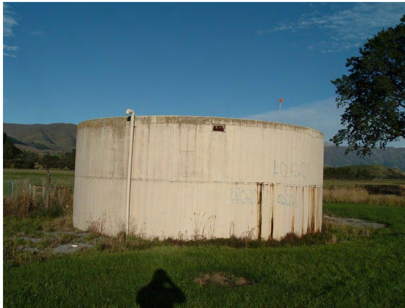
Figure 3.2.4a- Reservoir / Break Pressure Tank
