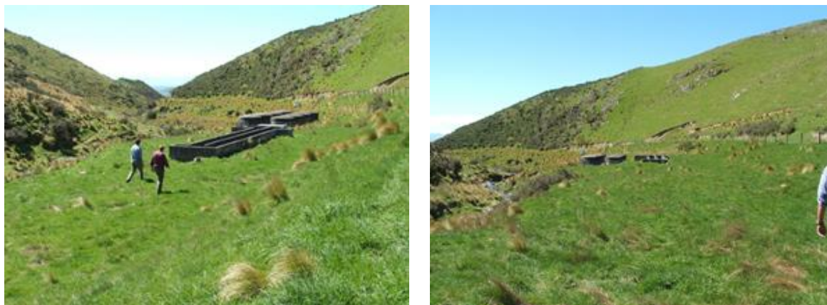
Figure 11-40: Albury WS Treatment Plant
