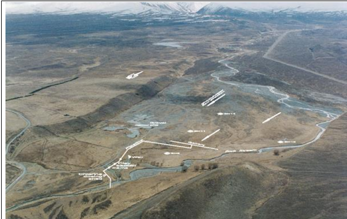
Figure 11-9: Lake Tekapo Water Supply Intake
