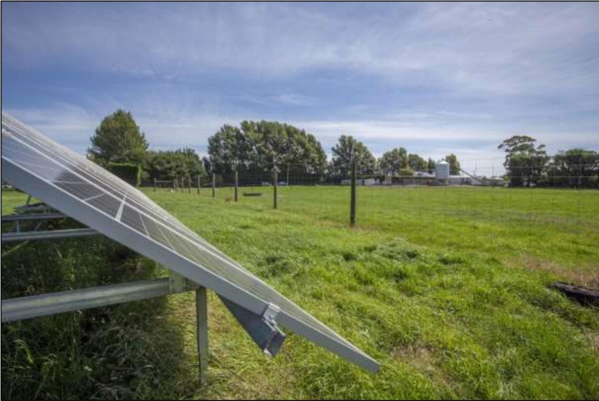
Figure 15: Another solar farm from the region – Keswick Farm Dairies Ltd, Rangiora. This photo shows that grass coverage over the ground does not diminish because of the PV modules. Please note that this module arrangement causes more shade than the proposed development at The Point, Mackenzie Country.
