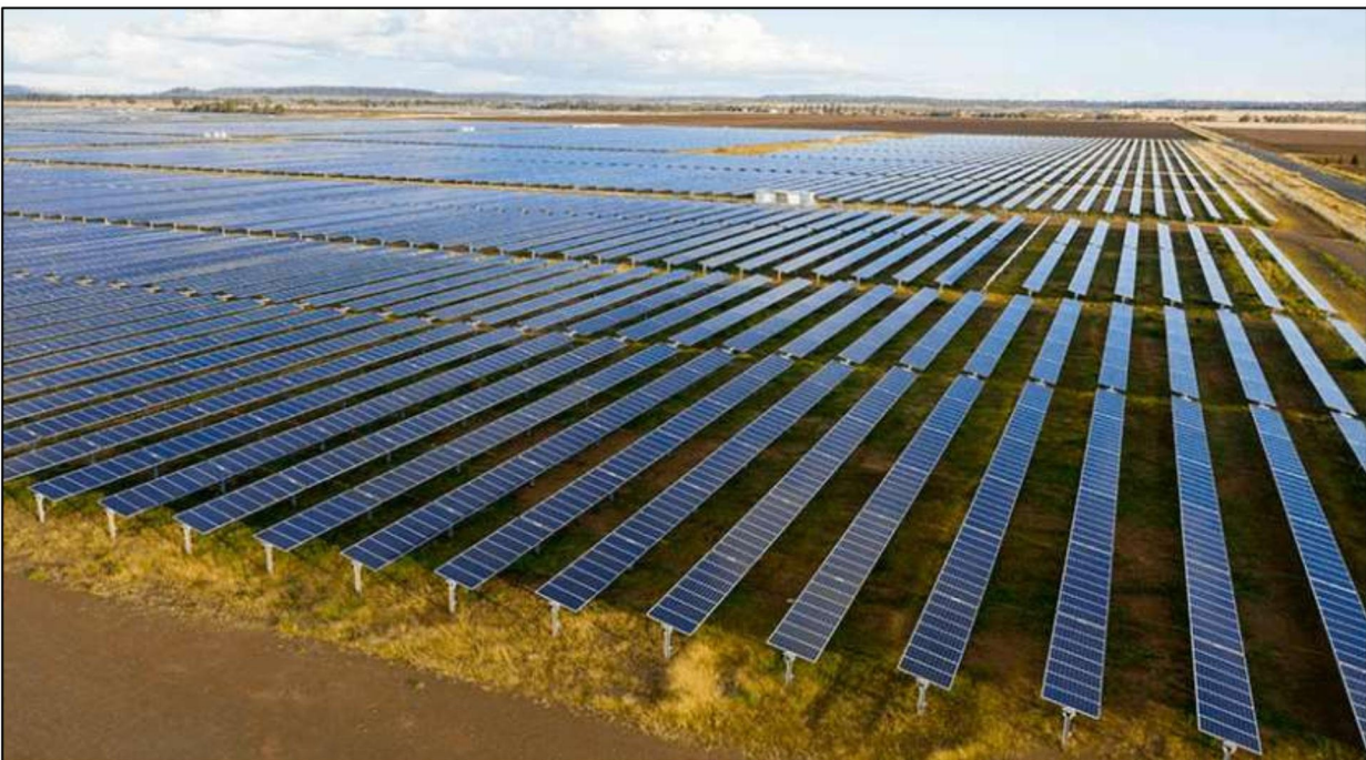
Figure 16: Solar Farm at the Pluto LNG Facility, Western Australia, demonstrates that grass coverage does not diminish in semi-arid conditions. This PV arrangement is similar to the proposed development at The Point, Mackenzie Country.
