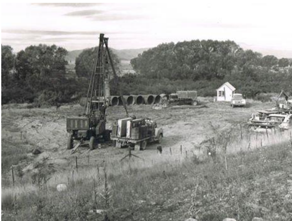
Photo: The original installation of the Twizel Water Supply wells.
