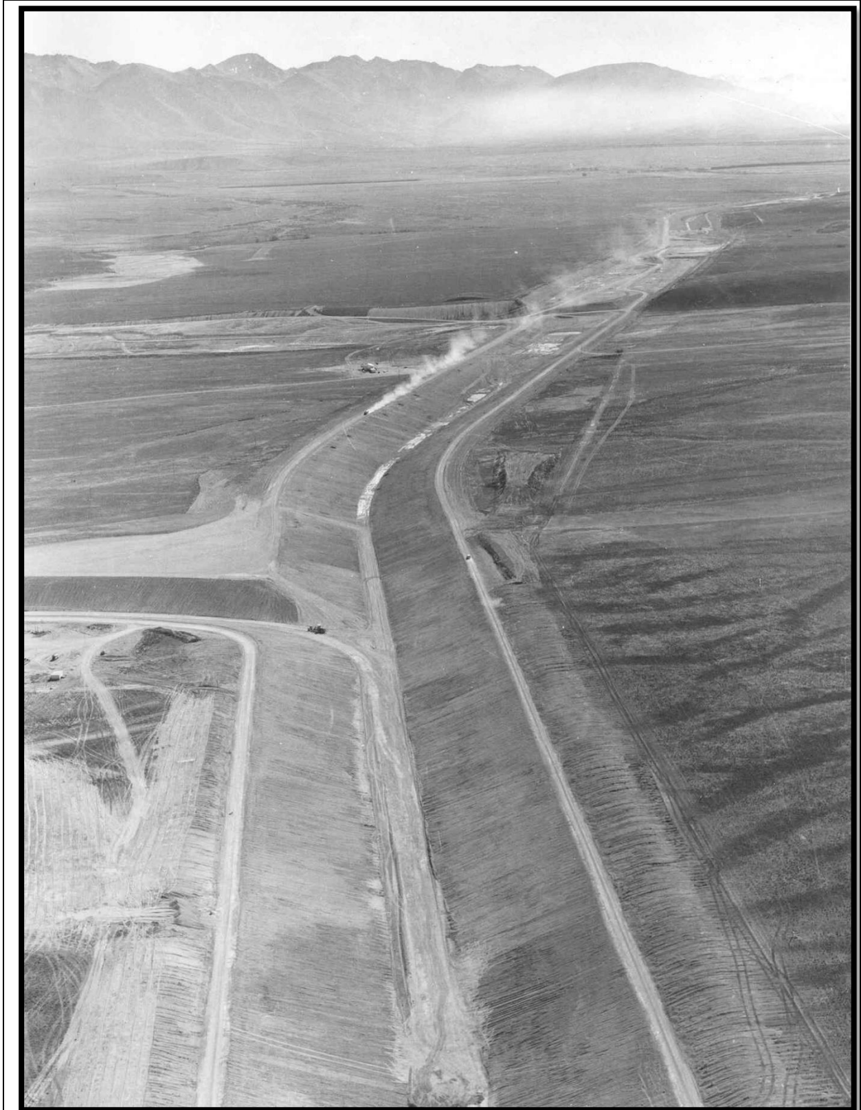
Photo 3: Work within the canal corridors, Pūkaki, Ōhau and Ōhau A canal junction. Photo taken looking upstream from the now Ōhau A Power Station during 1976.
