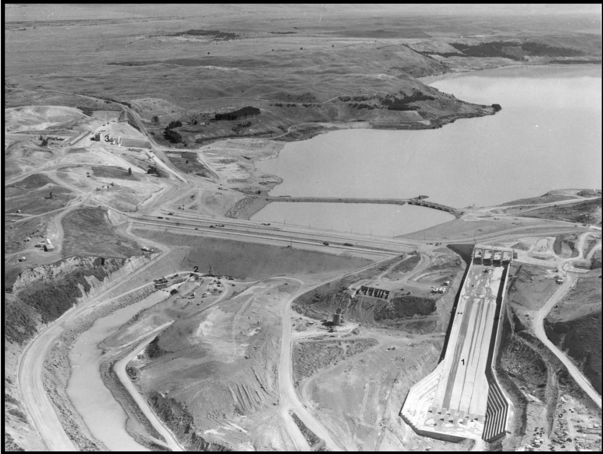
Photo 1: The working of the Core Land at the Pūkaki High Dam, when the High Dam was constructed in the 1970s
