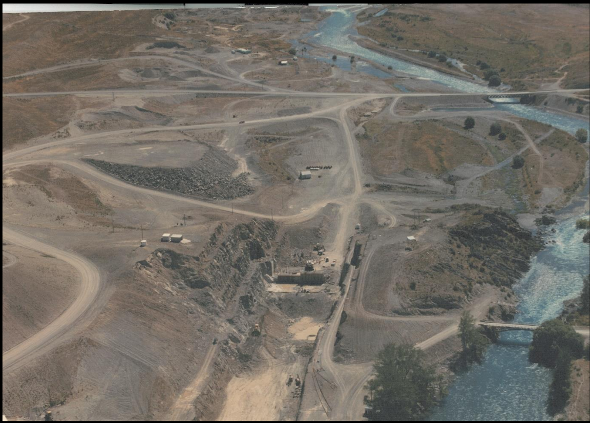
Photo 5: workings associated with the creation of the Lake Ruataniwha Dam and Control Structures - 1977
