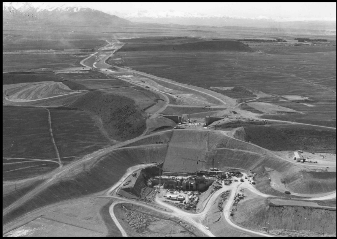
Photo 4: workings associated with the construction of Ōhau A Power Station – 1974.
