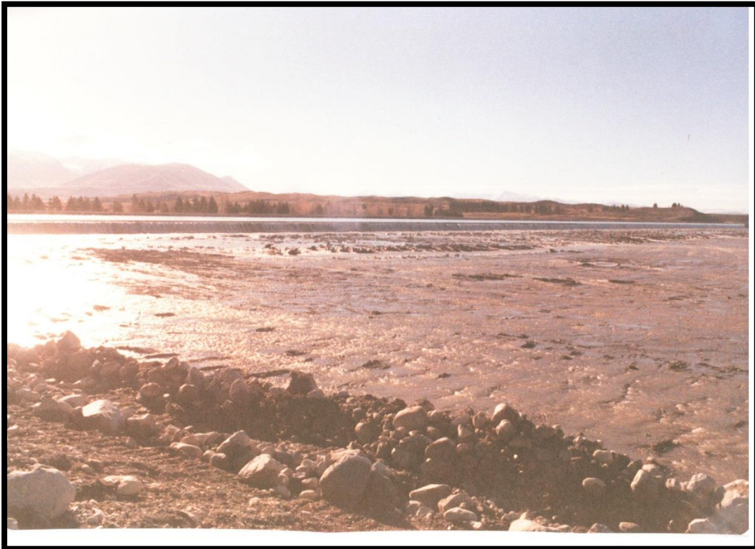
Photo 1: Pūkaki Canal topple blocks during 1979
