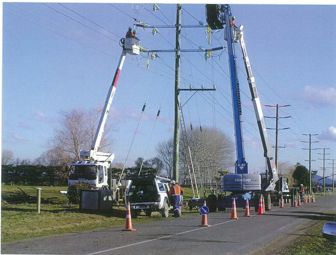
New distribution line to the Oceania Dairy Factory
