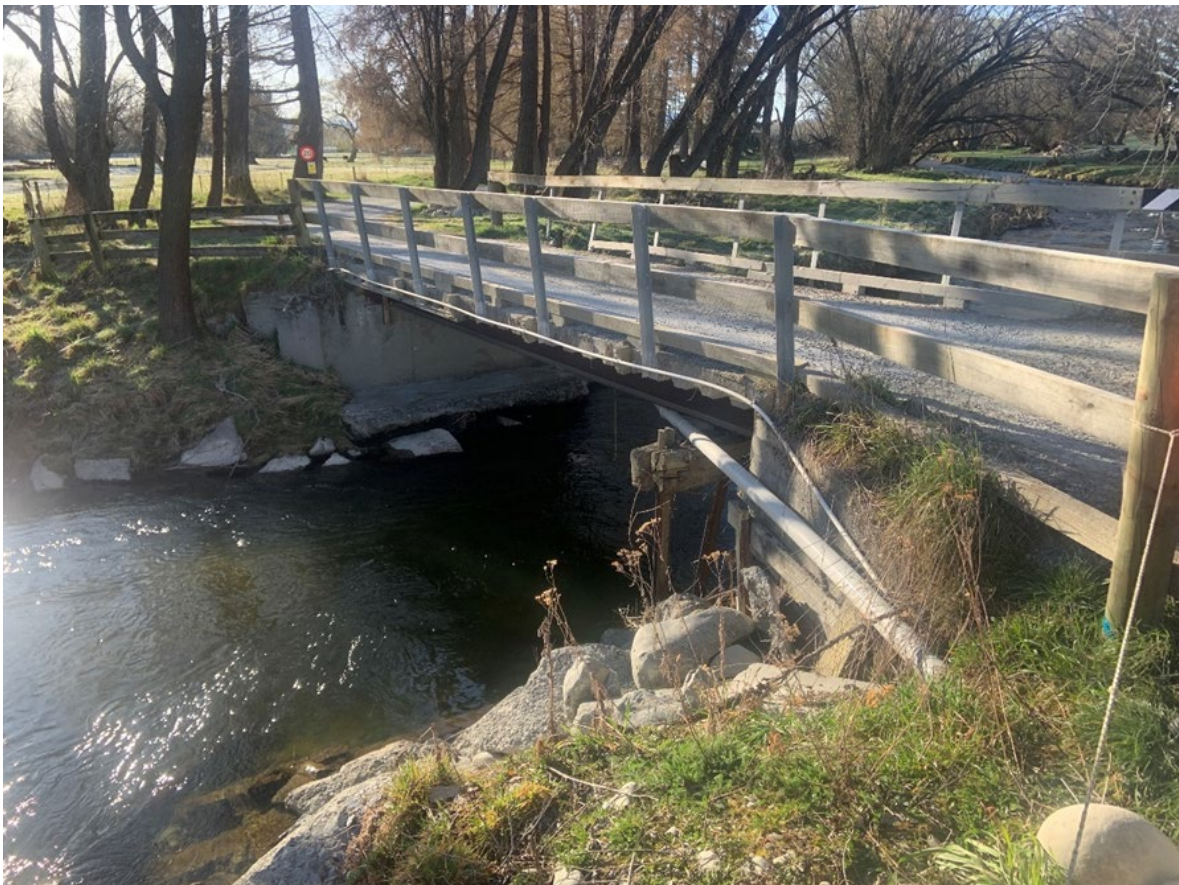
Figure 2 PVC pipe conduit used to carry the private pressure sewer across Frasers Stream (Bridge 1)
