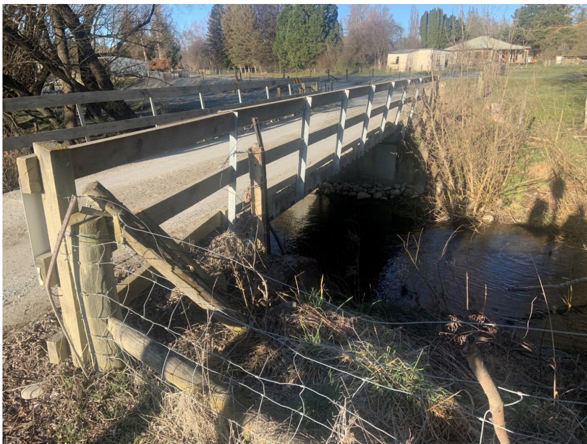
Figure 3 Dry Stream crossing (Bridge 2)
