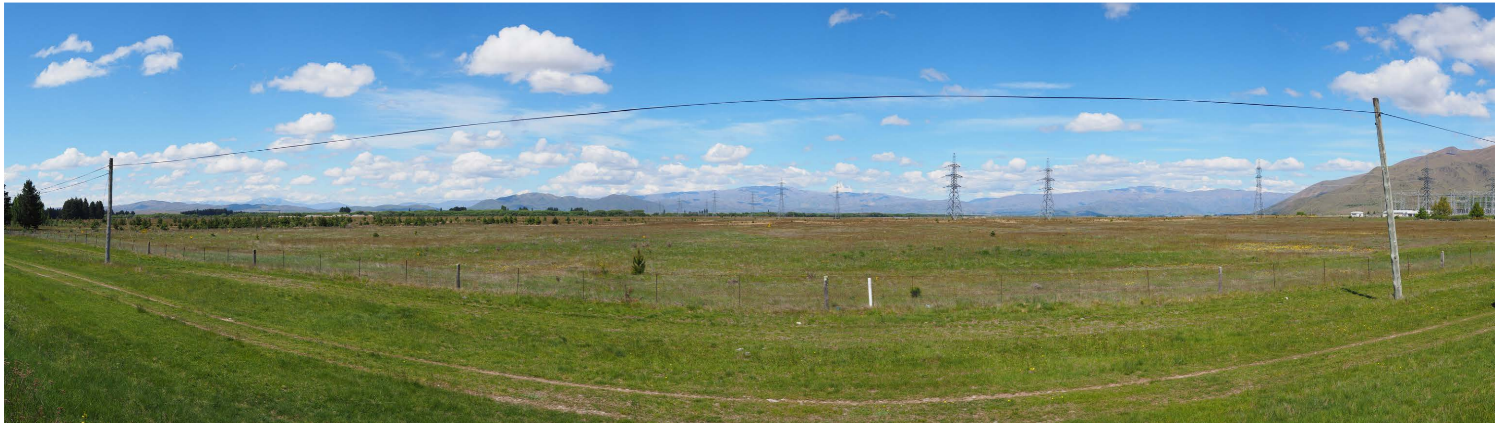
Viewpoint Location Photograph 2: Located near the Twizel Substation alongside SH8. This photo illustrates the view over the outwash plain towards the site and surrounding mountains, with the solar farm being 7.0kms away.
