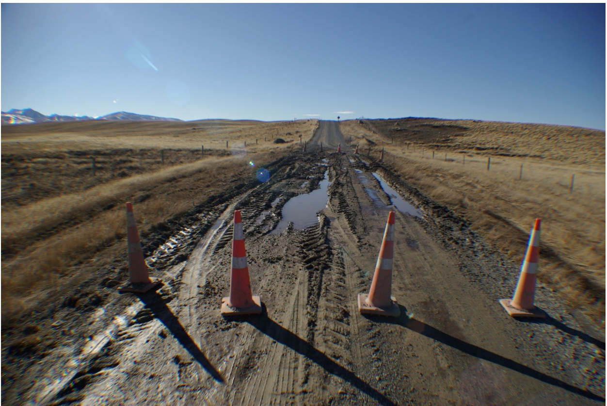
Real effect of frost heave on the Mackenzie District Council Network
