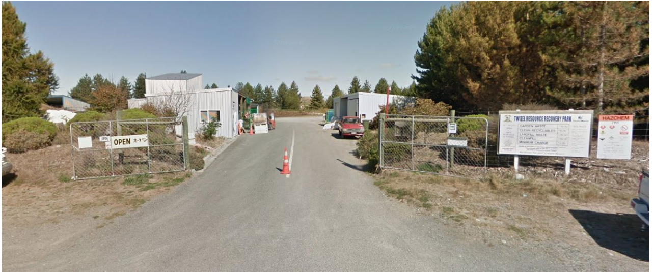
Figure 1: Twizel Resource Recovery Park at corner of Ostler Road and Hooker Crescent, Twizel
