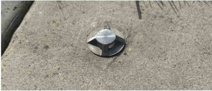
Figure 3 – Apron lights with a top shield. Source: Provided by the applicant.
