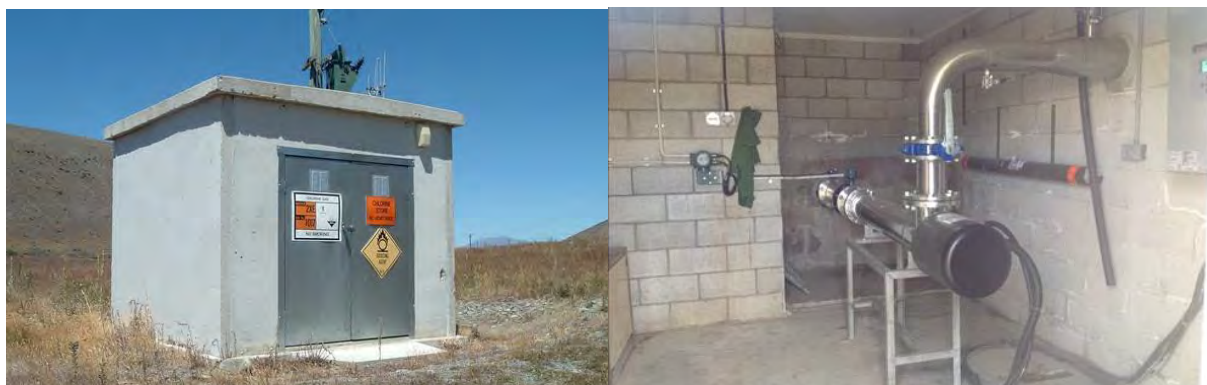
Figure 11-10: Lake Tekapo WS \text{Cl}_2 building & UV treatment
