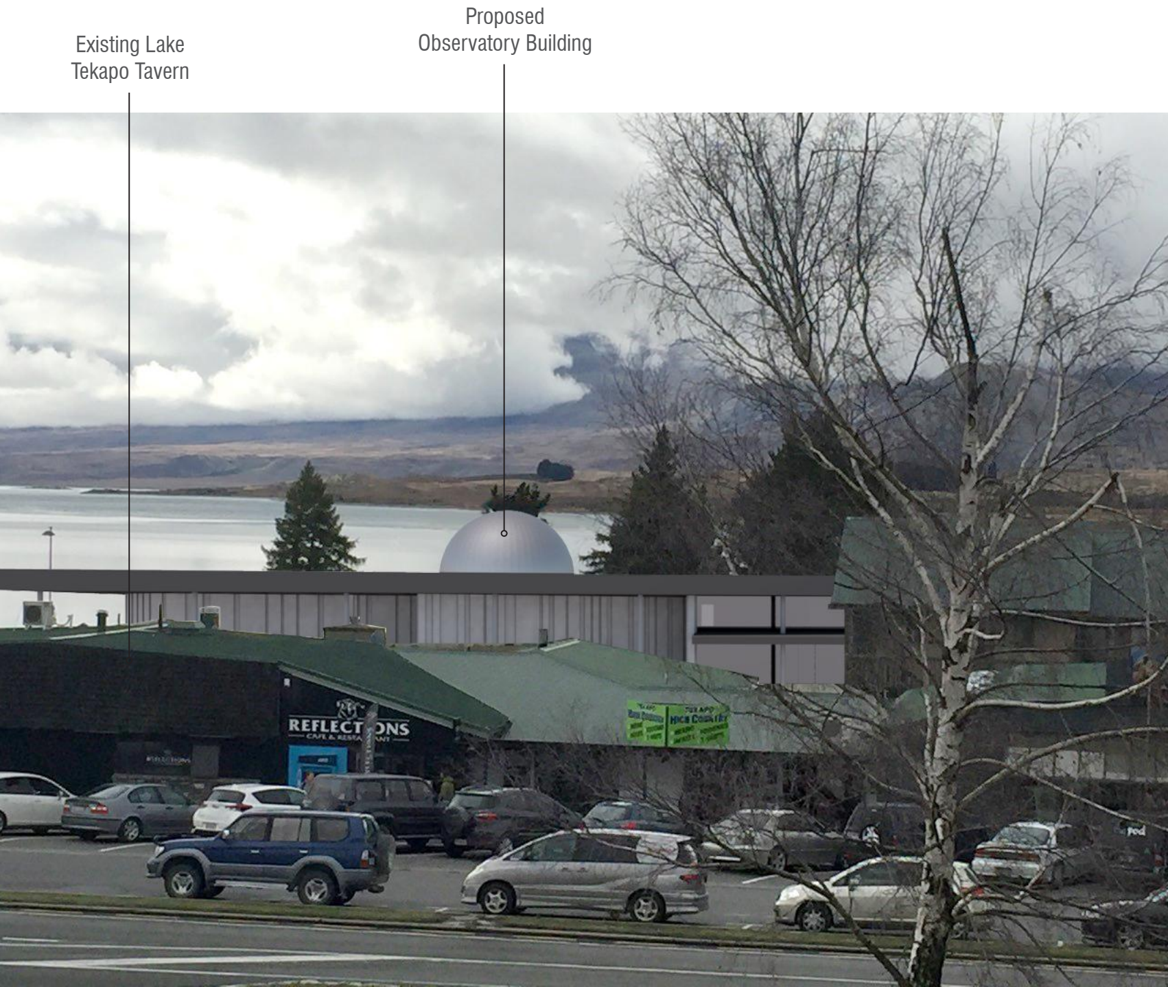
Figure-13 Image External View of Site (courtesy of Sheppard & Rout)
