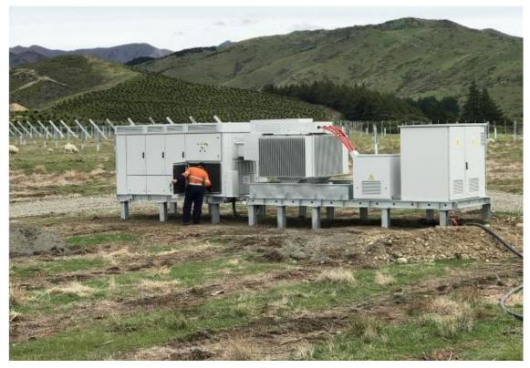
Figure 4: Photograph of HEMK MV skid gen 3
