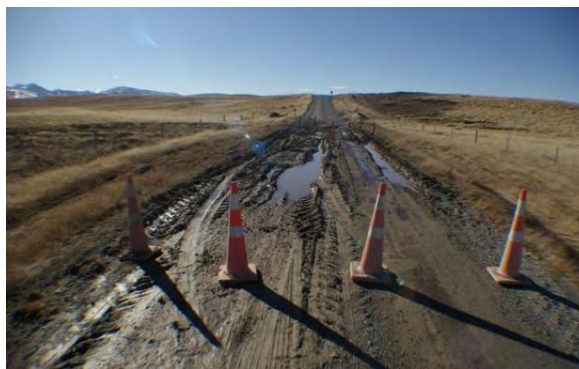
Braemar Road – Frost Heave July 2012
