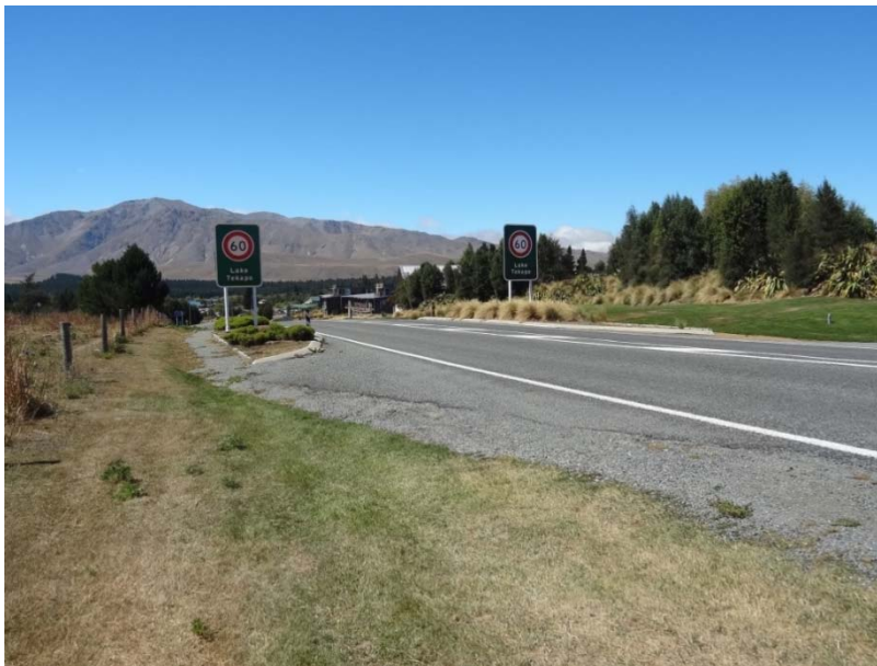
Photograph 1: Town Threshold Treatment on SH8
