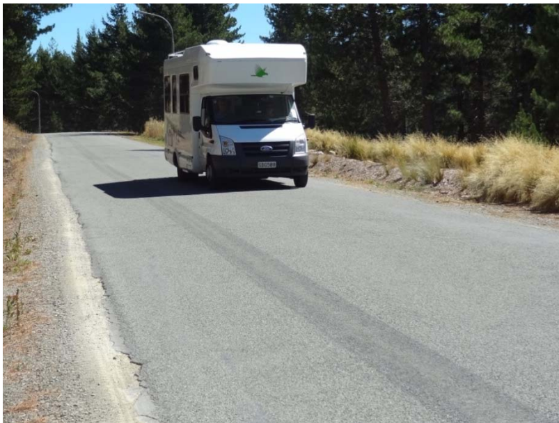
Photograph 3: Lakeside Drive – Shoulder Damage
