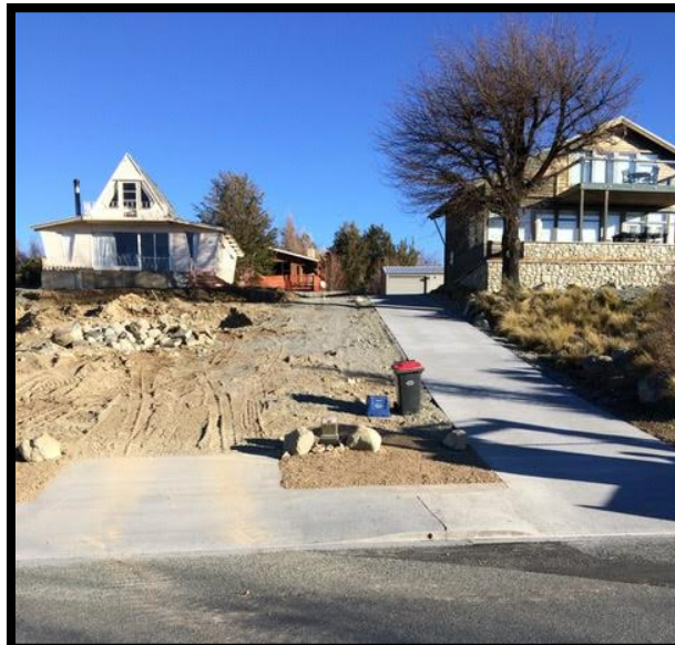
Figure 3 – The subject site in 2017 at the time of subdivision and prior to site development
