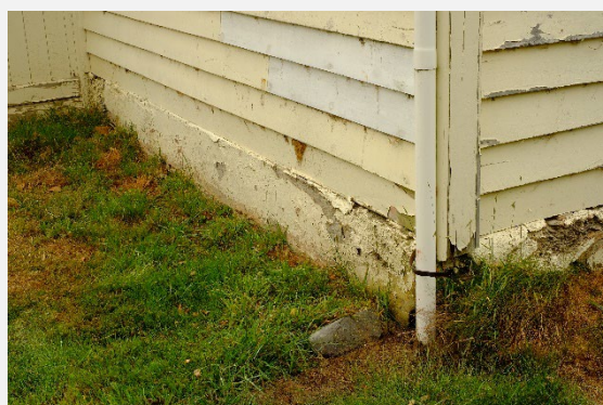
Figure 27: The building is set above ground level at the front, but at ground level by the rear of the lean-to (photo RKL 16 02 2024)
