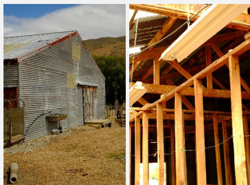
Figure 38: Bulging front elevation of woolshed and interior of woolshed (photos RKL 15 02 2024)
