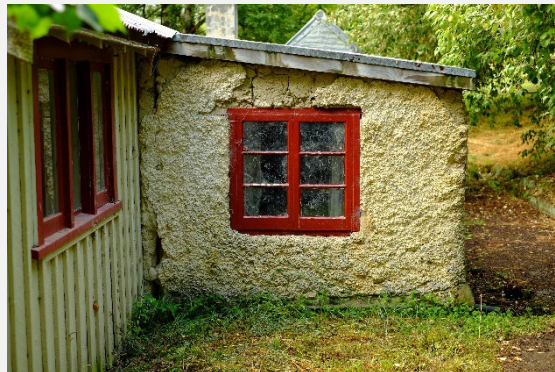
Figure 33: Cob lean-to at the rear (the other elevations of this are timber framed) (photo RKL 16 02 2024)
