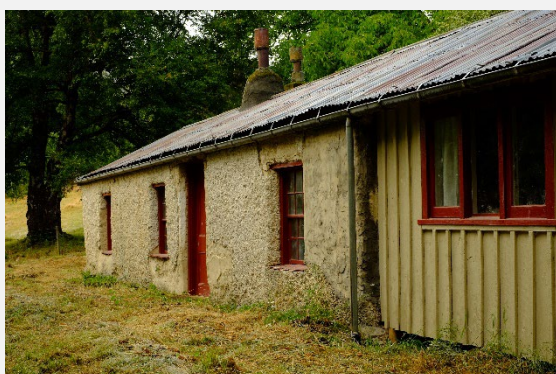
Figure 34: View along the front elevation of the building (showing the board and batten extension) (photo RKL 16 02 2024)
