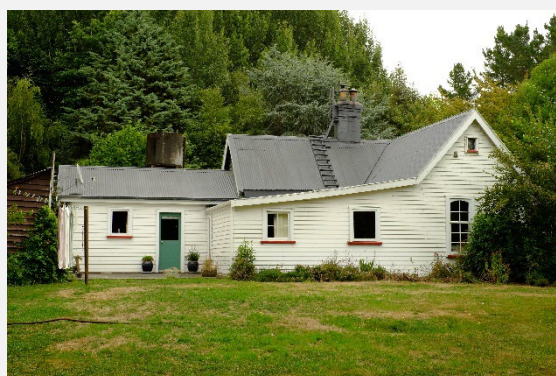
Figure 11: (top left) The building as existing, from the northwest. Note the altered cladding, altered windows in both elevations, and the lower pitch extension added on the south (photo RKL 15 02 2024)
