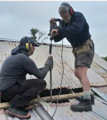
Council approved a grant for a partial contribution towards the earthquake strengthening of Anniss Cobb Cottage, Burkes Pass. The grant was used to purchase special screws designed for earthquake strengthening. One photo shows a sample of the 1.2 m Helifix screws used, and the other of one of the many screws being drilled vertically into the cob wall.
