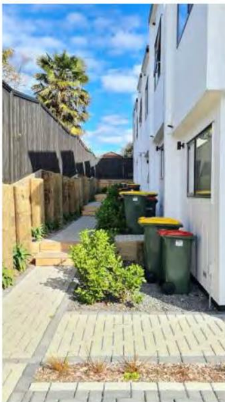
Figure 2: Bins areas without screens and stair access.
