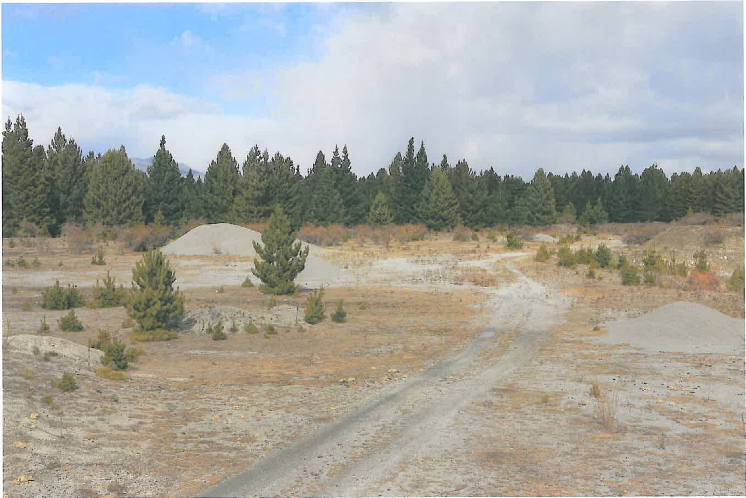
Figure 5: Derelict land, vicinity Loch Logan, Rhoborough Downs This area of borrow pits, stockpiles, weeds and compacted soils remains much as it was when abandoned at the conclusion of the Pukaki hydro development project.
