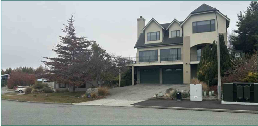
Figure 2: Photo of the dwelling taken from Hamilton Drive. Photo taken by B&A.
